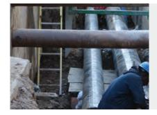
**HEATING OPERATION & TRANSMISSION DISTRICT, WASHINGTON, DC -** AFG provided PM and CM services on the underground Steam & Condensation Line Replacement Project for GSA for the project whole. The replacement of the lines, which serviced 21 government building sites, involved extensive amount of project coordination. Due to AFG's successful management, the project obtained substantial completion 93 days ahead of schedule.
