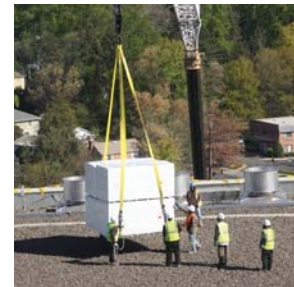
NIH Roof Repair
