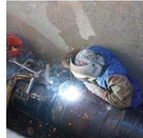
Steam Line Replacement
