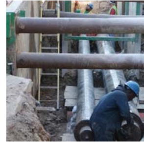
GSA Steam Line Replacement
