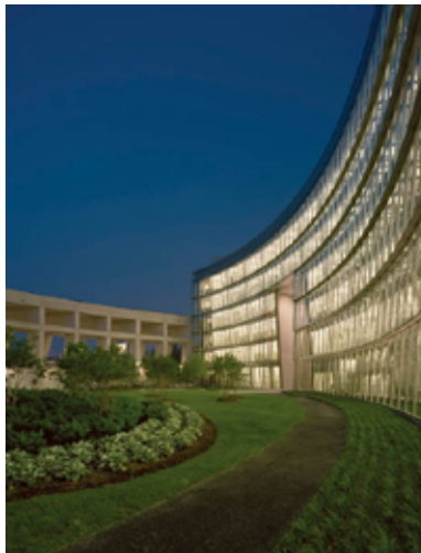
GSA National Deep Energy Retrofit 2 (NDER2) & Cx Program, Washington, DC
