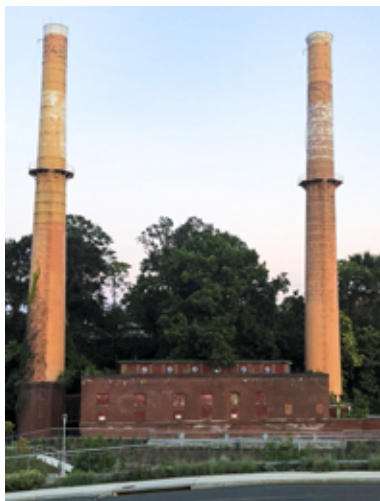
GSA St. Elizabeths Central Utility Plant (CUP2), Washington, DC
