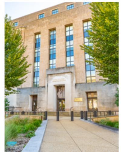
GSA Mary E. Switzer Federal Building, Washington, DC
