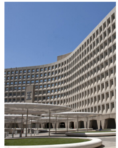
GSA Weaver Federal Building Fire Alarm Installation, $10M, Washington, DC
