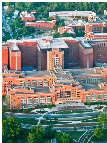
NIH Bethesda Campus, Various Fire & Life Safety Projects, Bethesda, MD
