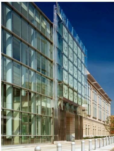
GSA Wheeling Federal Courthouse Fire Alarm Replacement, $1M, Wheeling, WV
